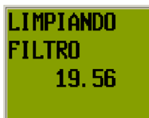
Photo: filter backwash screen.
